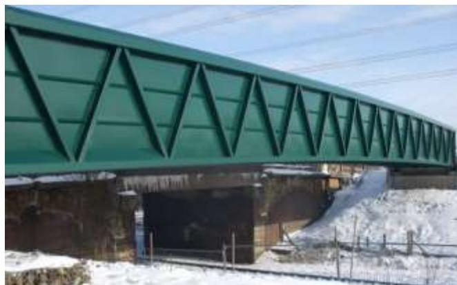
Figure 21: 32m fully clad footbridge over the railway between Halfway and Kilmarsh.
